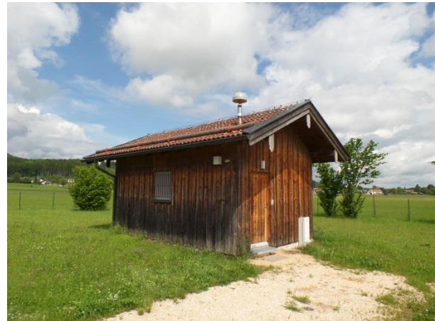
Neue Station Freilassing2
